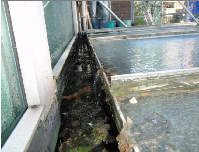
Figure 8 - Water testing of canopy.
