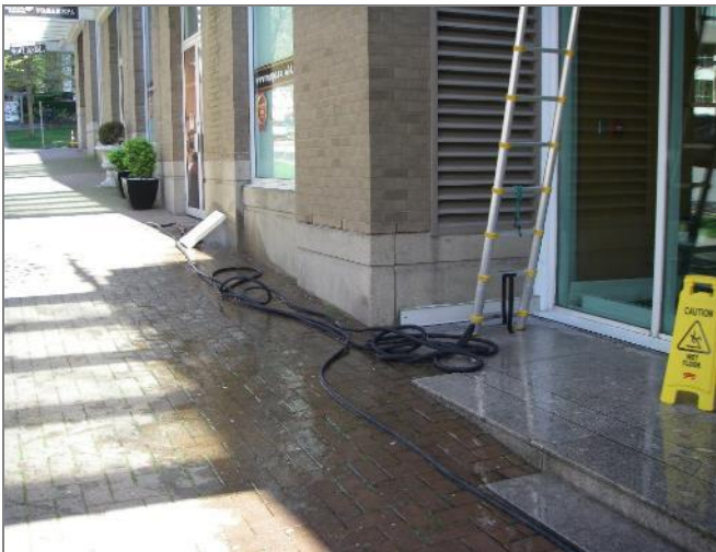
Figure 9 - Flood testing along sidewalk.
