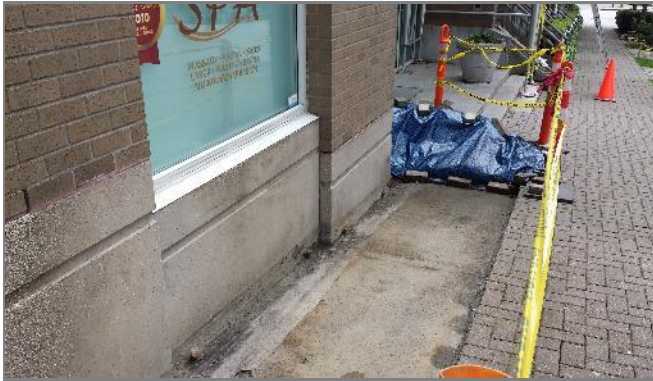
Figure 10 – Brick paving stones have been removed to expose the base of wall at west sidewalk.
