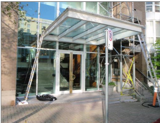
Figure 7 – Water testing at canopy.
