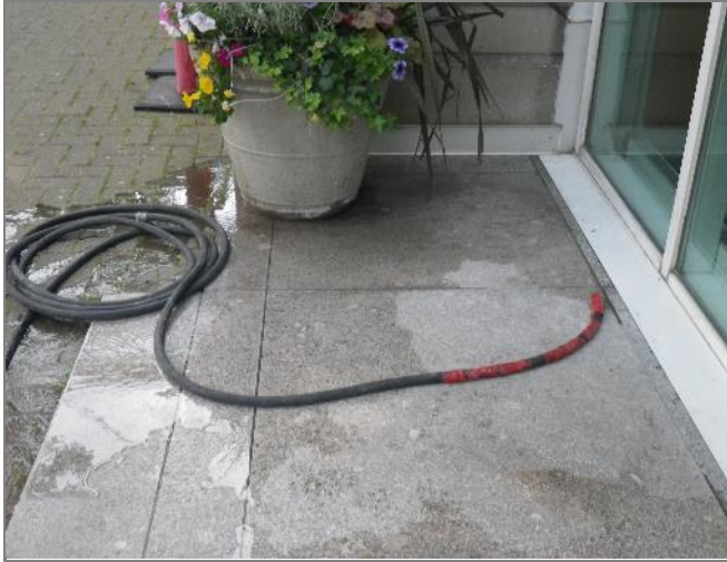
Figure 2 – Flood testing on granite tiles.
