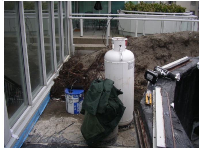
Localized repair at TH11
