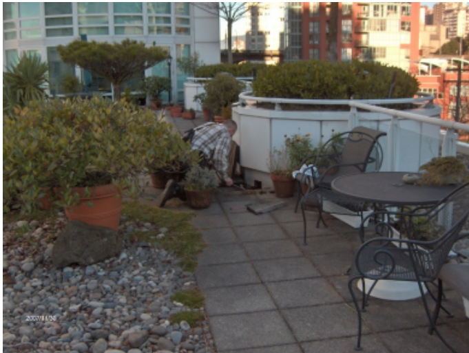
Localized repair at 711
