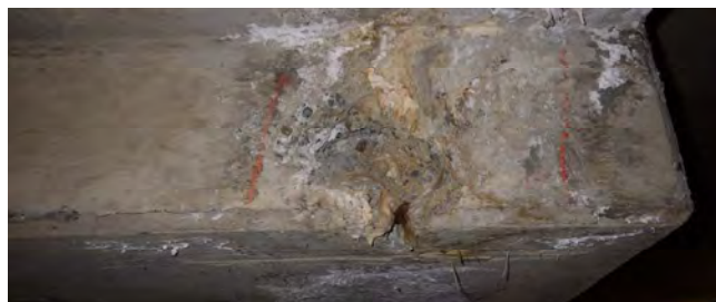
Spalling concrete
