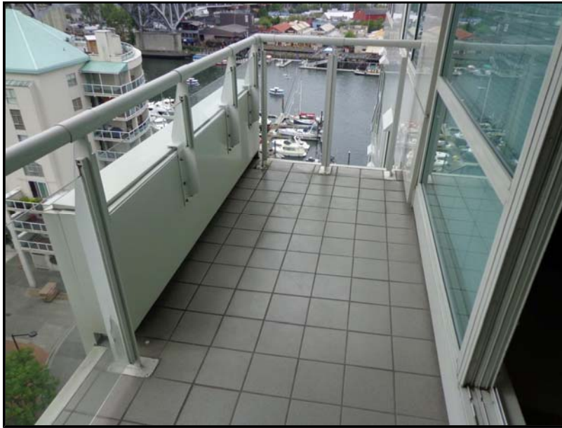
Photo No. 11: Balcony (Original tile at Ocean Tower. Others have elastomeric finish.)
