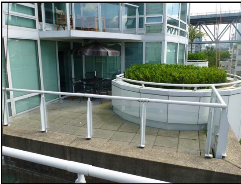
Photo No. 12: Rooftop terrace (typical)
