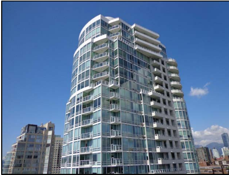
Photo No. 1: Beach tower - east elevation
