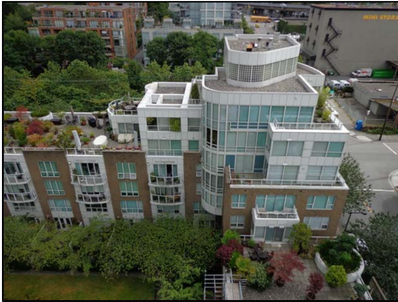
Photo No. 3: Garden Tower
