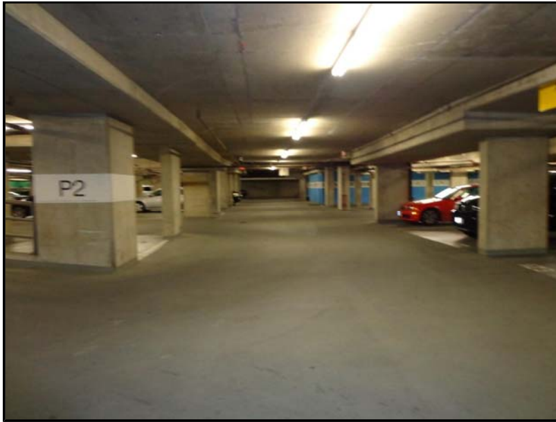
Photo No. 9: Underground garage
