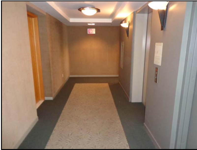
Photo No. 19: Tower corridor (typical)
