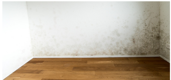
Condensation has led to mould problems on the drywall.
