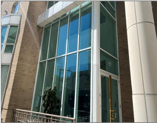
Figure 5.21 Curtain wall at Garden Tower lobby.
