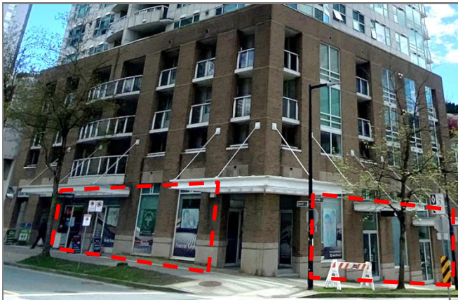
Figure 5.22 Storefront glazing at commercial suites adjacent to Beach Tower.
