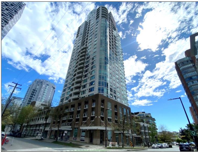
Figure 2.2 Beach Tower, as viewed from the northwest.
