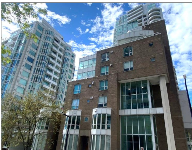
Figure 2.3 Garden Tower, as viewed from the east.
